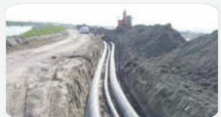
Sprinkler main pipe installation
